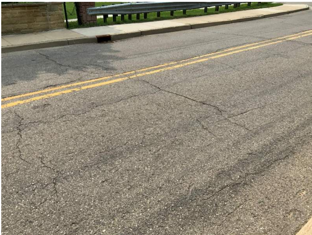
Cracks in wearing surface
