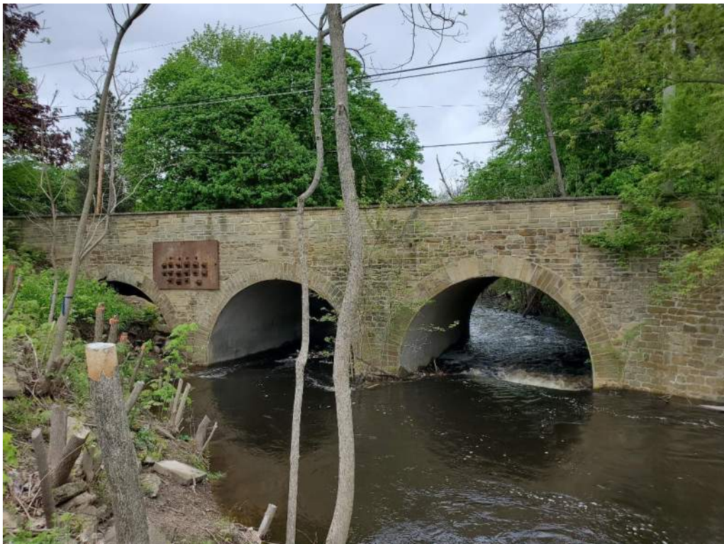
Upstream elevation, south culvert blocked, steel plate repair
