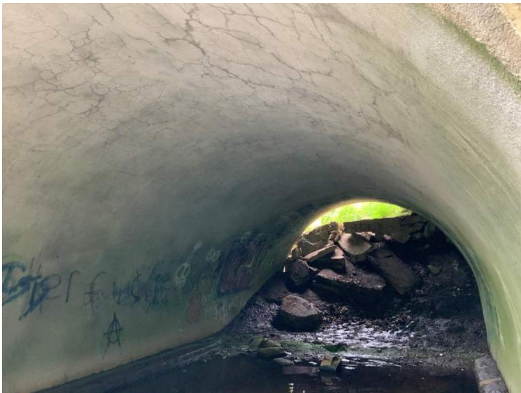
Upstream face of the south arch intentionally blocked
