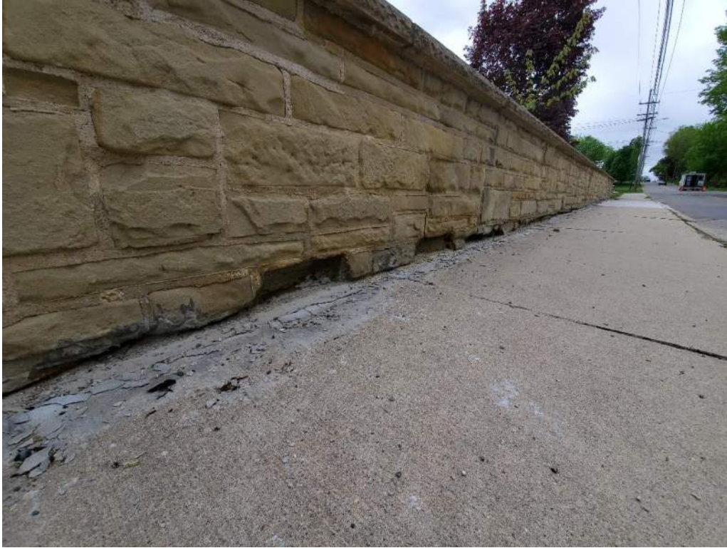
Deterioration along bottom of railing allowing infiltration along headwalls
