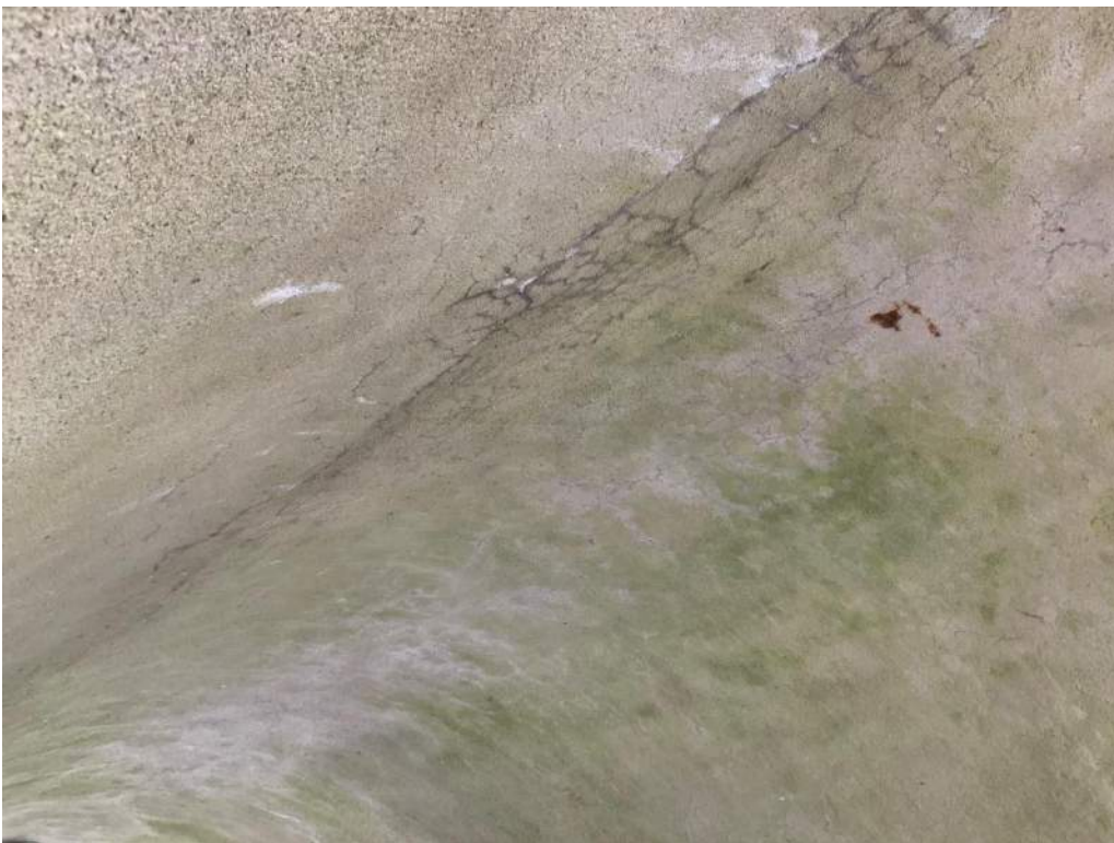
Cracks with efflorescence in bottom of arch
