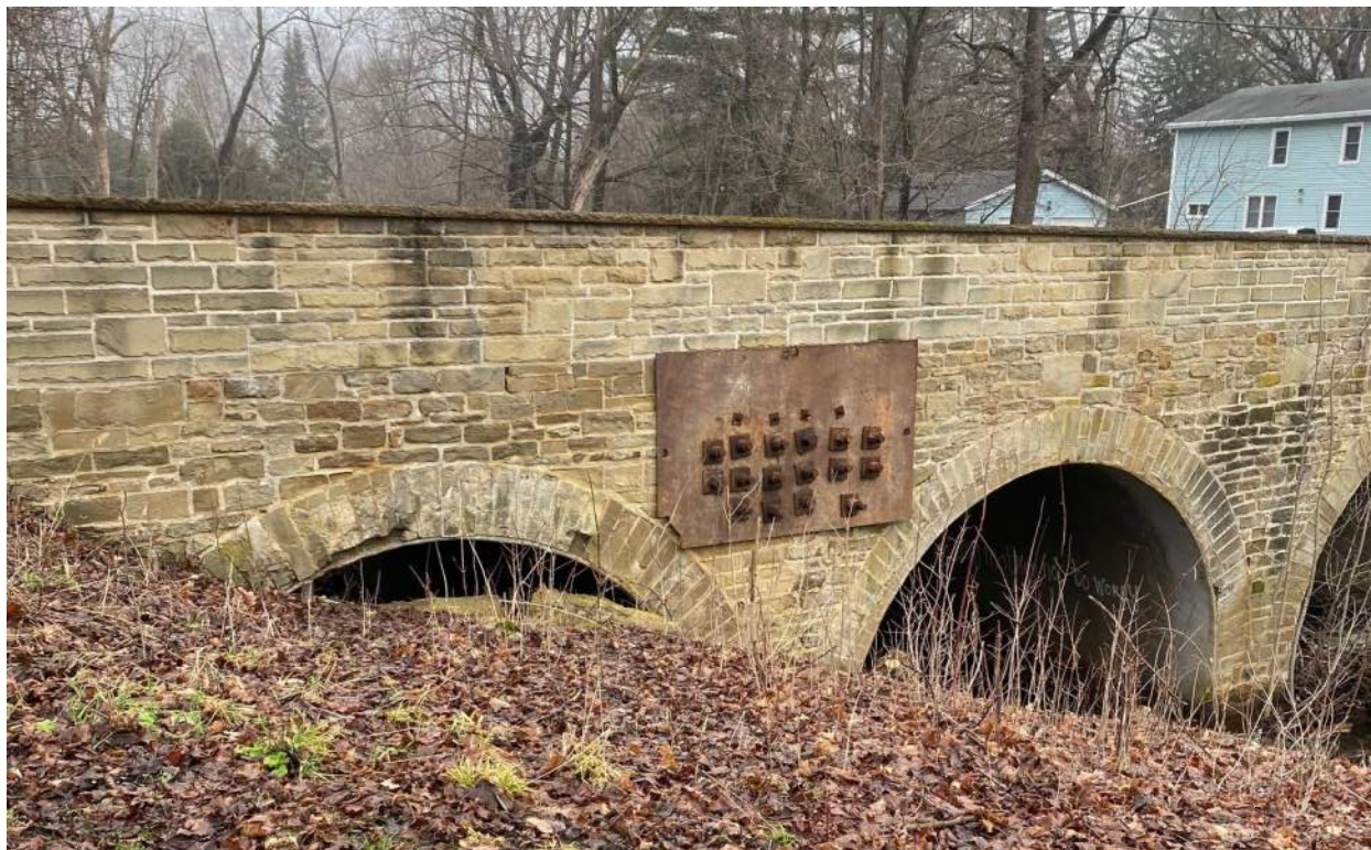
Steel Plate repair on east headwall
