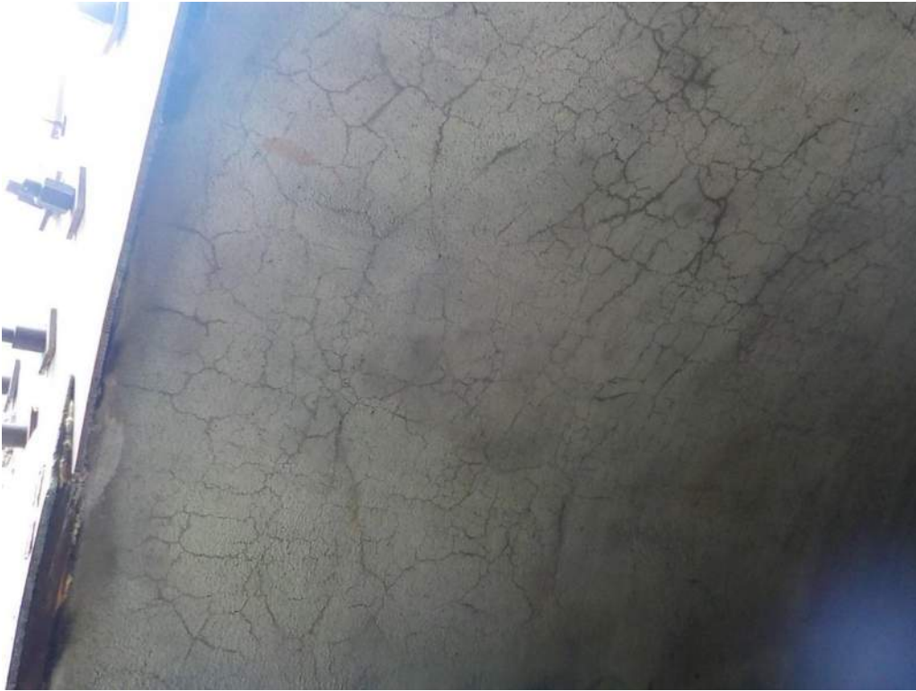
Cracks in bottom of arch
