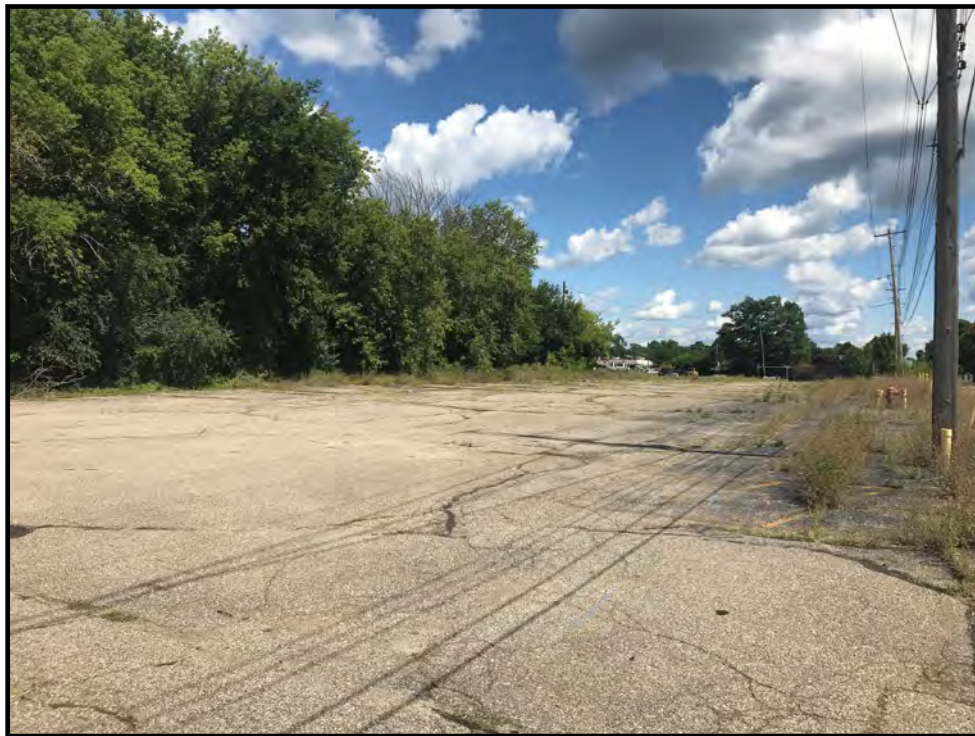
Photo 2: View of the Property to the northeast from the southwest corner of the Property.
